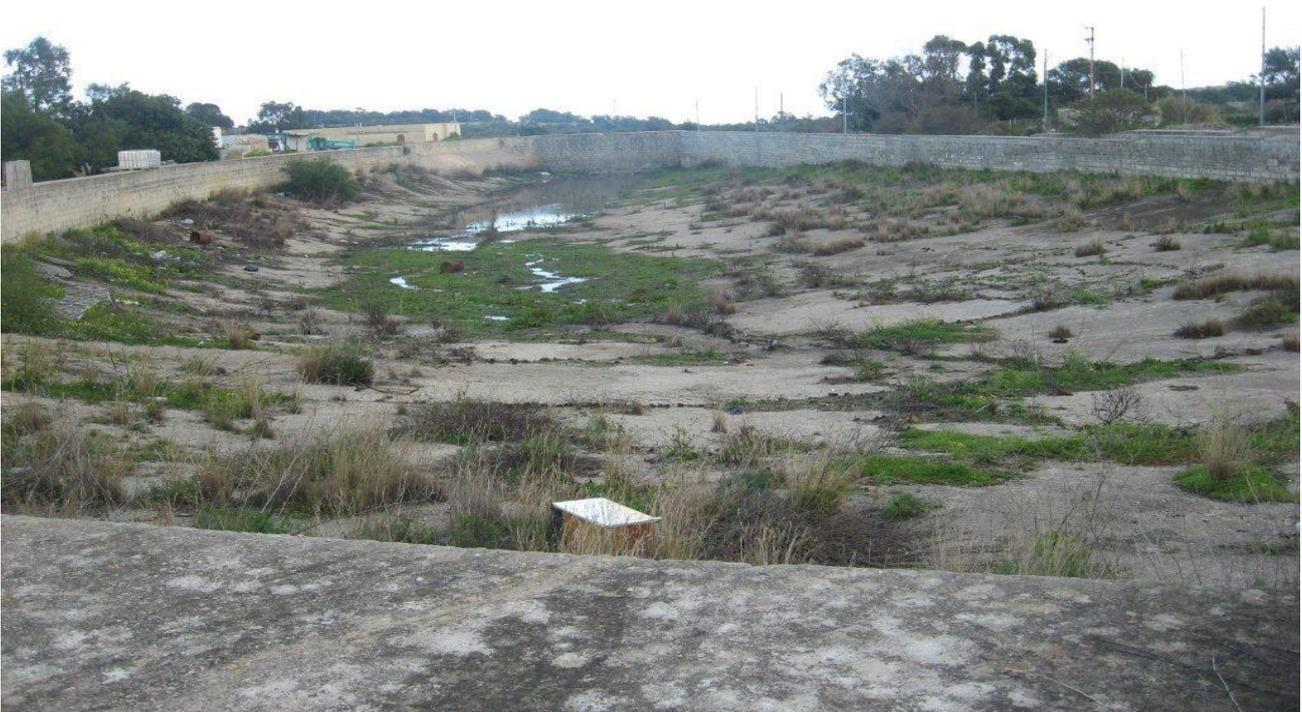
This reservoir was built in 1977 when the new runway was constructed. Its purpose is to collect the rainwater that falls on this runway. This reservoir has a capacity of 70,000m<sup>3</sup>. From information provided by Eng. Marco Cremona, this reservoir loses water through leakages therefore it is not in use anymore.
